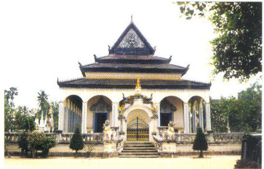
Figure 1: Vat Bo Pagoda, vihear seen from west
